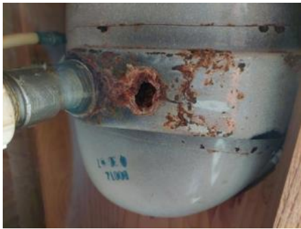
Bottom of bathroom sink
