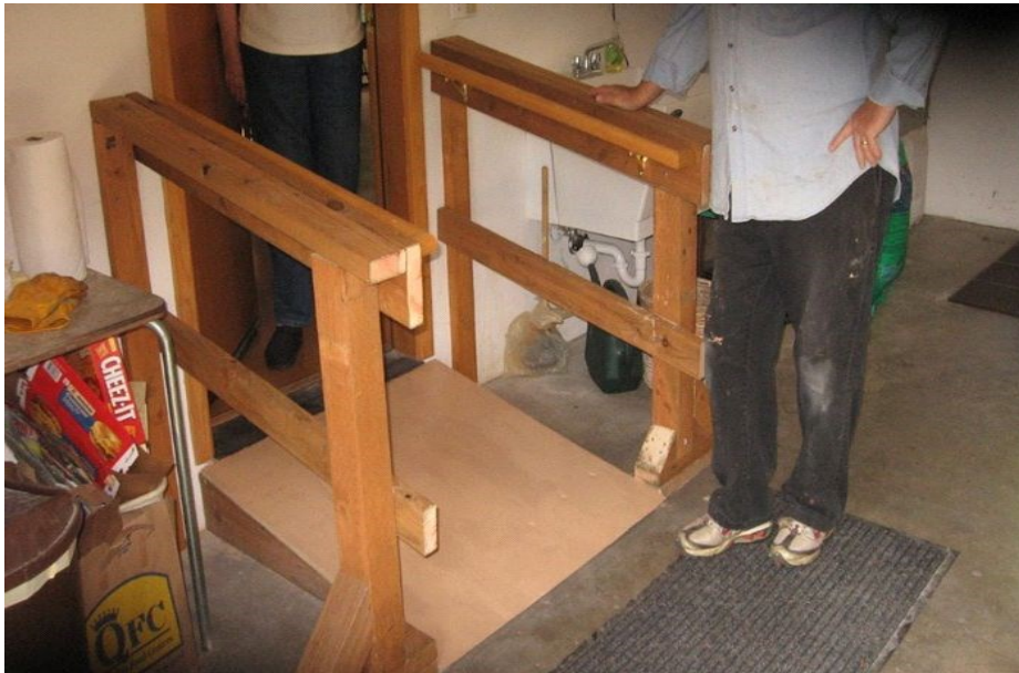
Railing with Ramp
