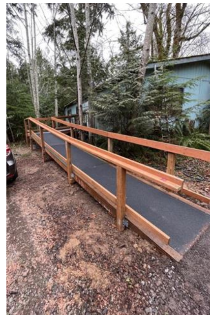
Ramp at its new location in South Kitsap.
