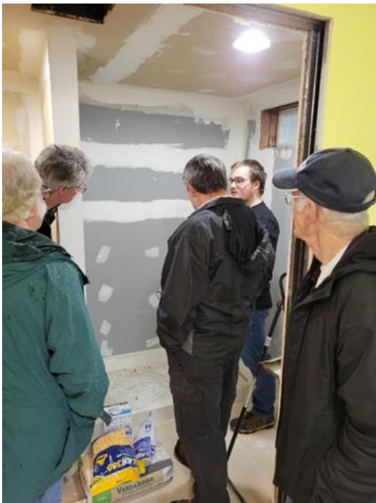
Lot B – during repairs
