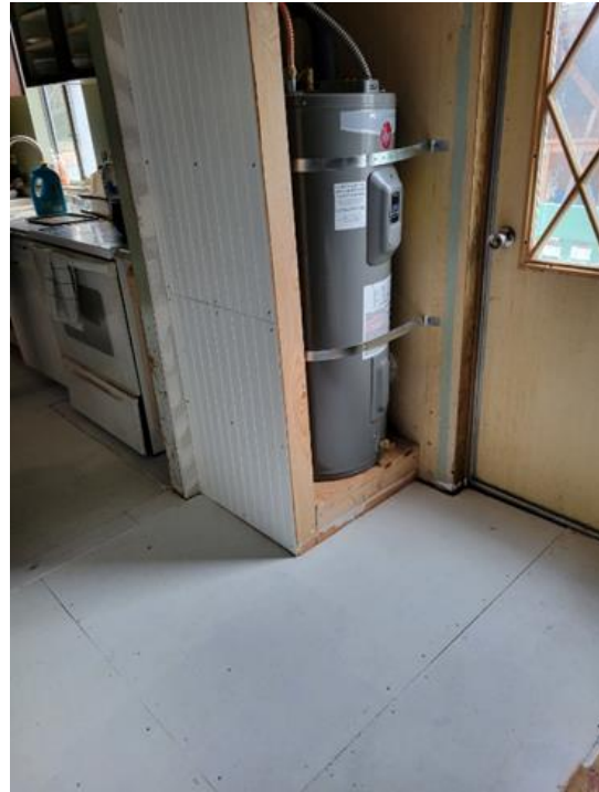
Lot A – after repairs
