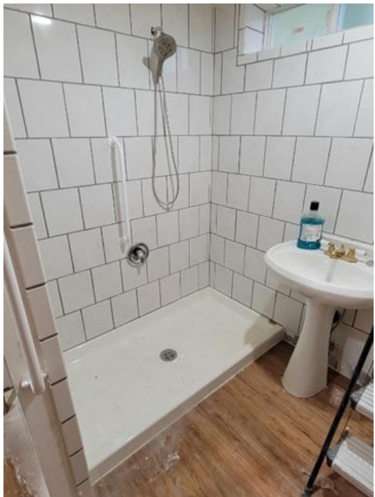
Lot B – after repairs
